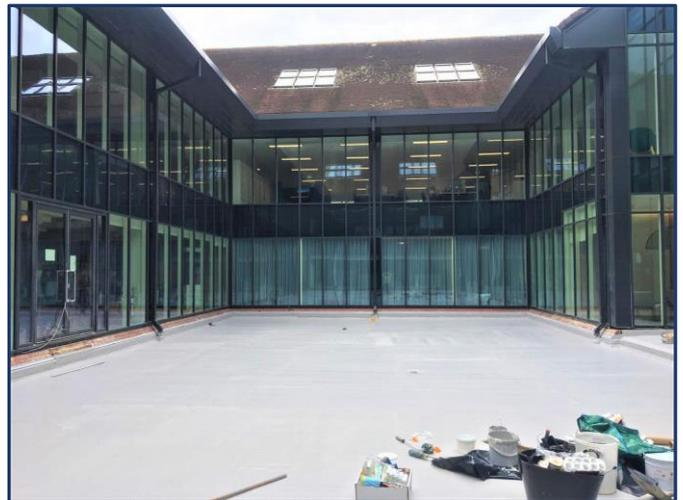
The PremDeck goes on in two layers. The first is a resin with fibre mat combination with another layer of resin above the top. Then comes the finishing topcoat which dries hard but allows some flexibility from the fibres.
